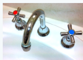
Photo 2 Cross head taps that are colour coded will enable a person with dementia to easily identify and use them.
