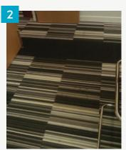
This principle can also be applied to other floor surface areas such as steps, escalators and lifts. Choosing materials that reduce the colour contrast but still achieve the desired outcome is possible with careful consideration. Australian standards require raised tactile floor surfaces to assist visually impaired people. If these are done in a solid dark colour, it can create the perception of a large hole for someone with dementia. Using a sensitive design tile can avoid this.
